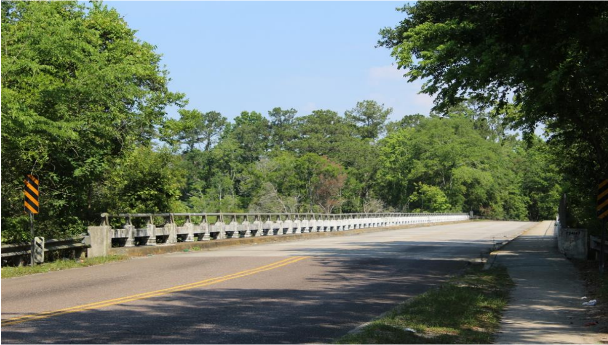
Ribault River Bridge, pre-construction
